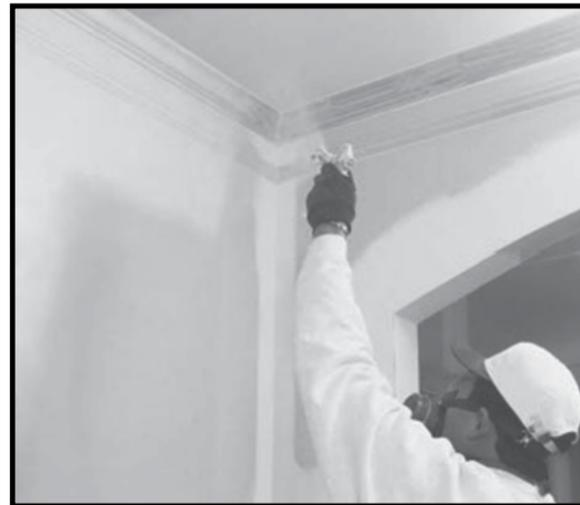
Turn down the pressure as low as it can go while still spraying a good spray pattern to reduce your tip and pump wear. Turning down the pressure also saves paint by reducing overspray.
